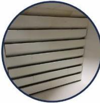
*The Element are fitted into neat Element Grooves that are manufactured into the kiln walls, this provided a snug fit, elements are less likely to come out and they are protected from possible damage from packing and unpacking of your kiln.*
